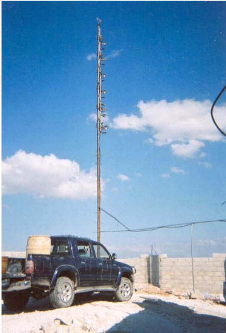
COMPLETED ANTENNA WITH LINE SUPPORT STRUCTURE
